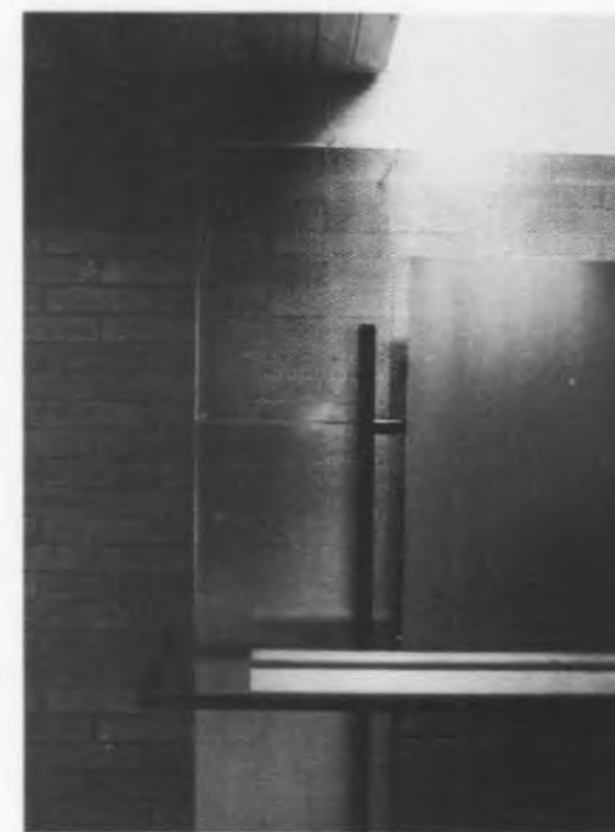
Above: detail at top of stair showing careful assemblage of materials: fir plywood panels, fir handrails, and perforated aluminum screens are fixed on painted steel channels. Above right: section through spine showing the skylight slot which brings natural light to the interior of the gallery.
