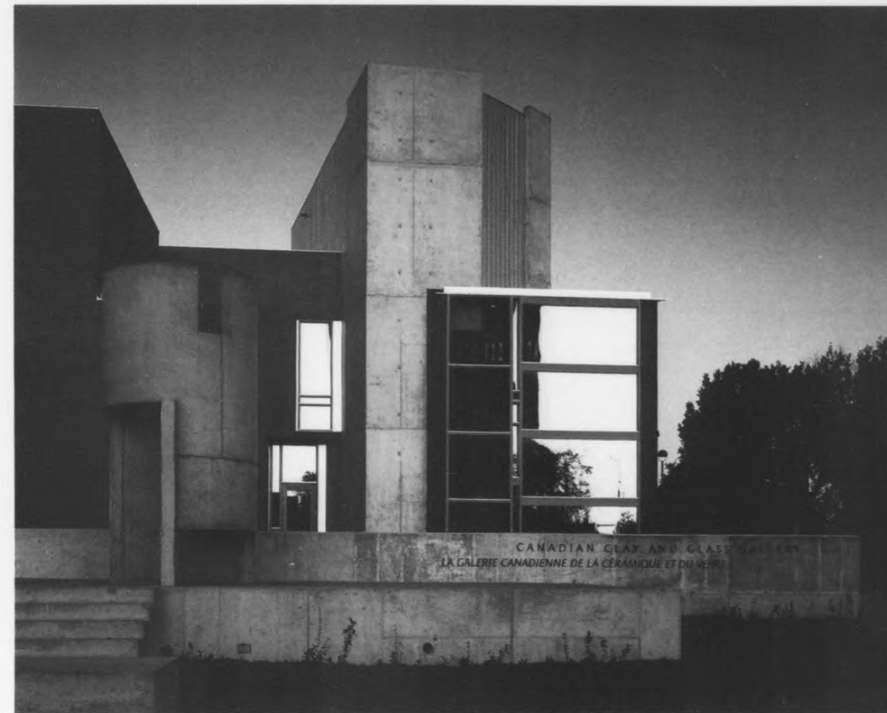
A heavy triangular mass known as the Tower Gallery hinges prow-like off the north end of the uniform red brick envelope.
